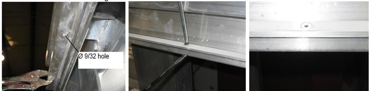
7. Insert the white nylon track insert in the lower track flush to the track ends and temporarily hold with vice grip.
