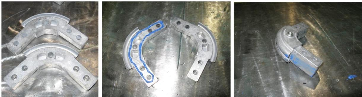
2. Install corner assembly and clean away excess silicone.
